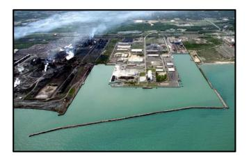
The rubblemound breakwater is the harbor's only protective structure. Three sections, totaling 600 feet overall, require repair work.
